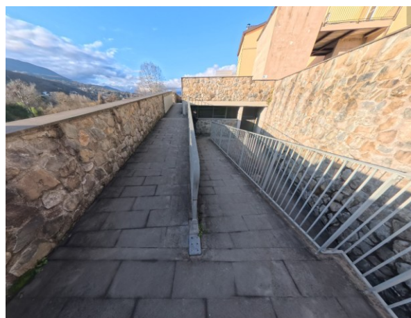
29 Ramp connecting elevator – Theater
