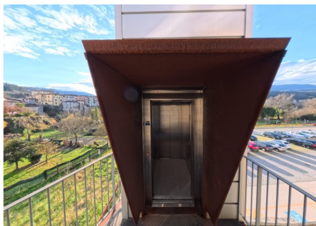
28 Elevator connecting the Theatre car park – ramp
