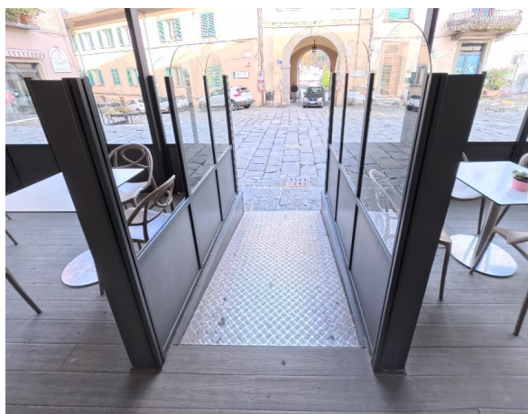
38 Ramp for Bar access
